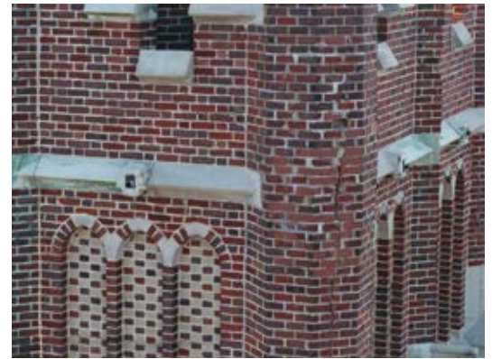
Figure 3. Drone head-on close-up image of deteriorated masonry.
