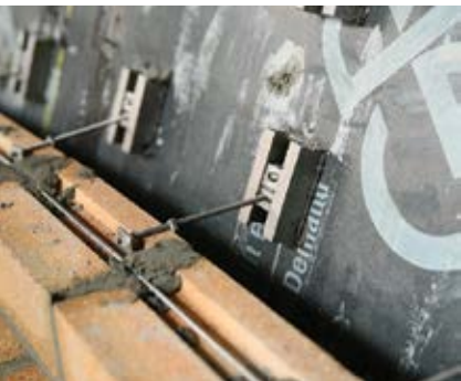
Figure 4. The custom brick tie system.
