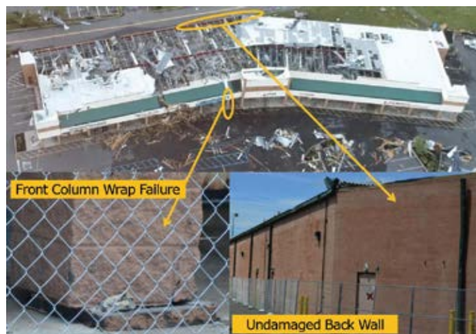
Figure 3. Building B overall damage; typical front column wrap shear failure in mortar joint (left); back wall of building undamaged (right). Aerial photo from 570 Drone footage.
