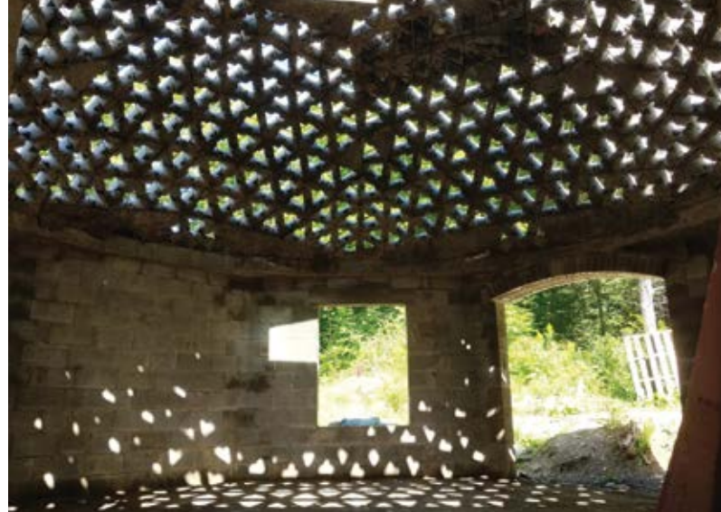
Masonry dome made with manufactured concrete block by Spherical Block LLC.
