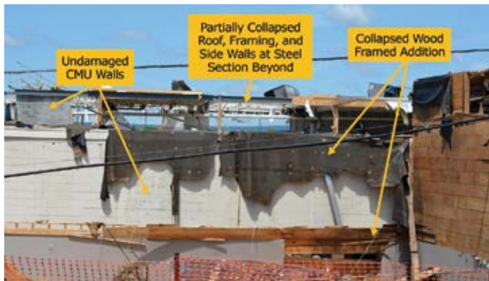
Figure 2. Building D (middle and background) and Building A (foreground) partial collapse of wood and steel framed elements in line with undamaged CMU walls.
