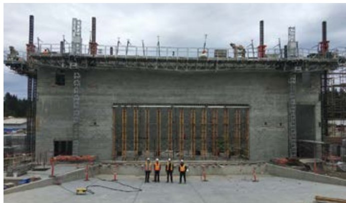
Elevation of the CMS wall and beam during construction. Approximately 40 feet of 60 feet completed.
