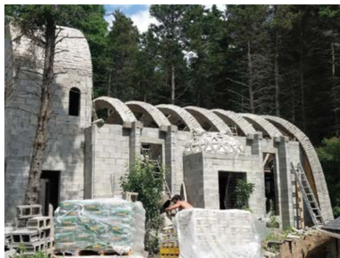
Masonry arches and flying buttresses made with interlocking block by Spherical Block LLC.
