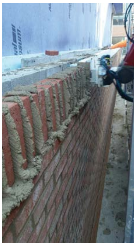
Semi-Automated Mason (SAM) by Construction Robotics.
